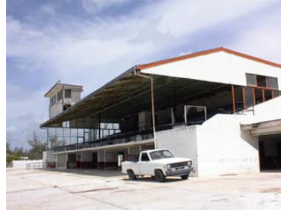
Asbestos testing at Old Dog Track, Stock Island
